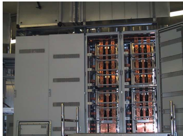
1,5 MW Converter for wind power plant (Vensys 70/77)
