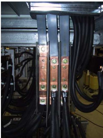
1,5 MW Converter for wind power plant (Vensys 70/77)
